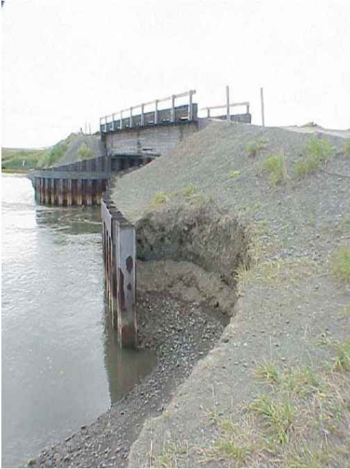
Photo 1 : Erosion at the Tununak bridge that connects to the airport, 2003.
