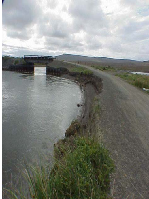
Photo 2: Erosion of the road to the airport, September 2003.
